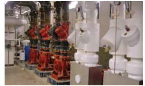
Chilled Water & Condenser Water Pumps
