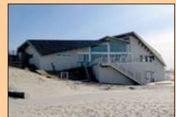
Construction of Dockweiler Youth Center was completed.
