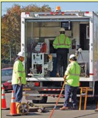
Workers assess condition of sewer line.
