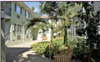
The CDC rehabilitated an existing apartment building into the Alexandria House Apartments, consisting of 16 studio and one-bedroom units (seven of which are reserved for homeless families).
