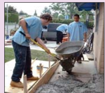
Youth workers participate in a home rehabilitation project.
