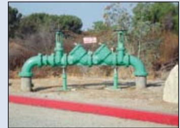
Santa Fe Dam Fireline and Transformer
