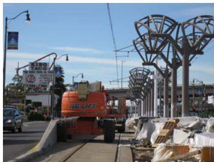
Gold Line Eastside extension Maravilla station under construction as of December 2008 with King Taco in the background
