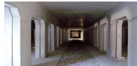
A view of the infiltration system recently constructed below Sun Valley Park.
