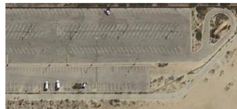
Image 29: Lack of turn around
