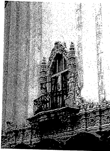
Figure 3.2-2 Balcony Above Primary Entrance
