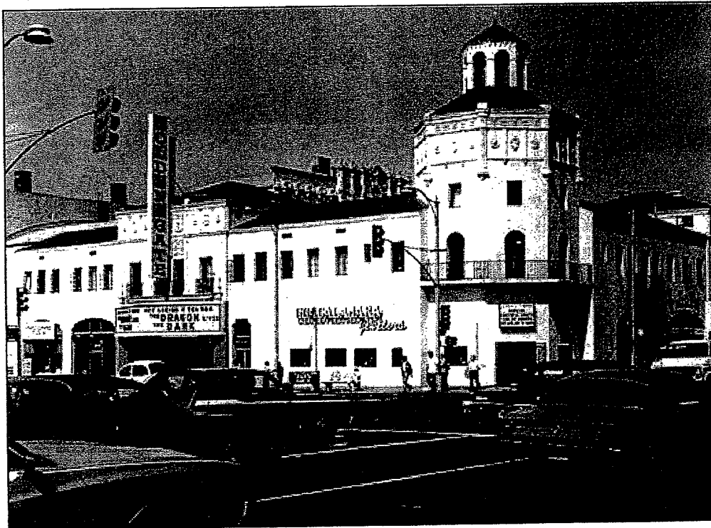
Figure 4: Golden Gate Theater, view southwest, (upper portion of north façade visible) wrapped by the Vega building (demolished) (William Reagh, Los Angeles Public Library Photo Collection, Photo No. 0015322, 1980)
