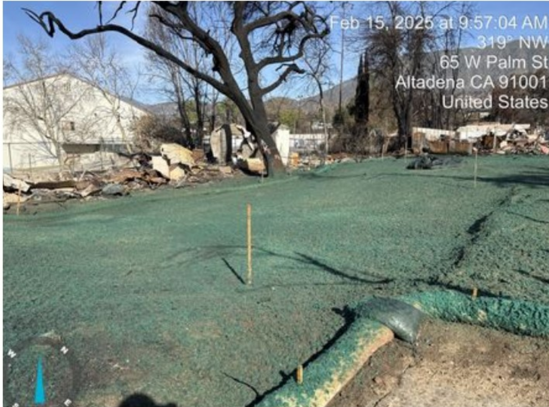
Picture 7: Example of appropriate level of erosion control with hydro-mulch (Eaton Fire 2025). Erosion Control must be implemented to prevent sediment runoff.
