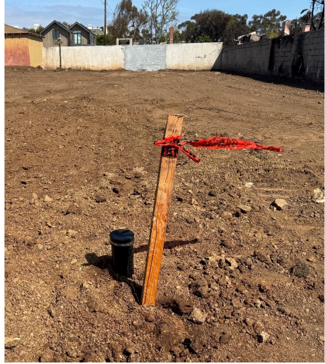
Picture 1 & 2: Examples of capped sewer lines. Stake or flag the location of the sewer line on the property.
