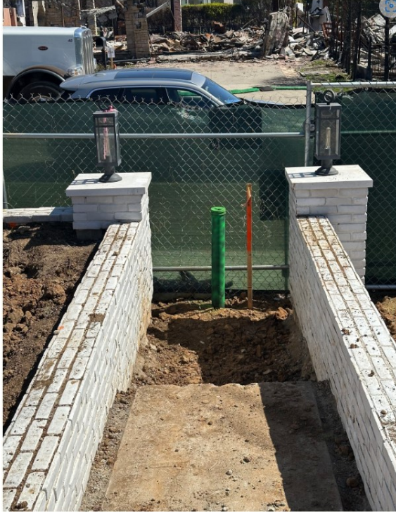
Picture 1 & 2: Examples of capped sewer lines. Stake or flag the location of the sewer line on the property.
