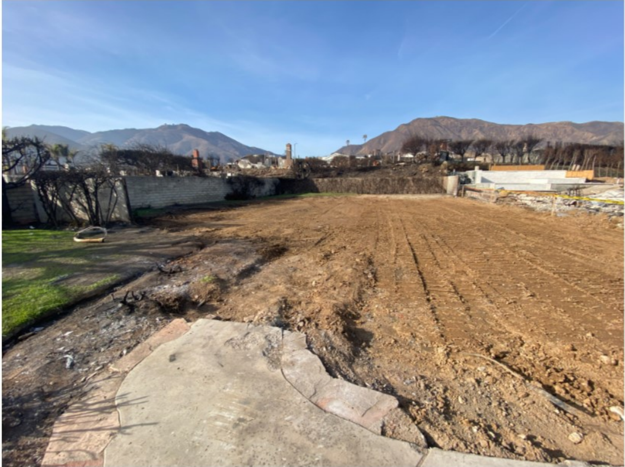
Picture 5: Example of appropriate level of soil removal and foundation clearance (Palisades Fire 2025). Erosion Control will be implemented to prevent sediment runoff.
