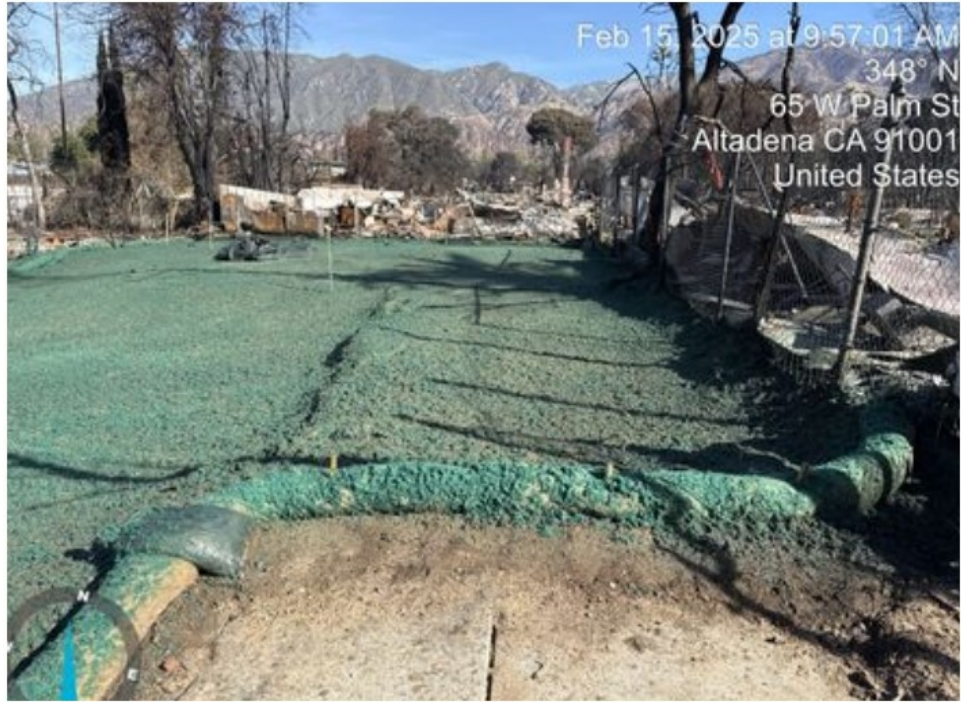
Picture 4: Example of appropriate level of erosion control with hydro-mulch (Eaton Fire 2025). Erosion Control must be implemented to prevent sediment runoff.
