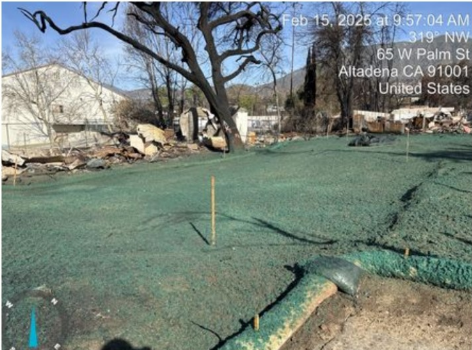
Picture 4: Example of appropriate level of erosion control with hydro-mulch (Eaton Fire 2025). Erosion Control must be implemented to prevent sediment runoff.
