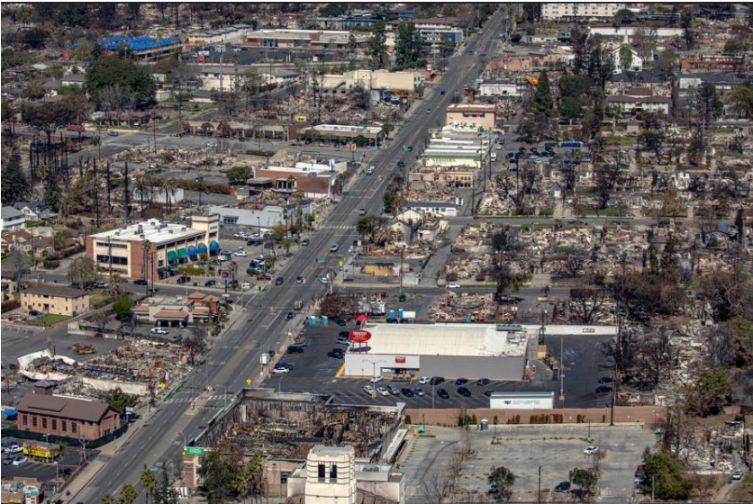
Aerial photography of damages to businesses in Altadena 2
