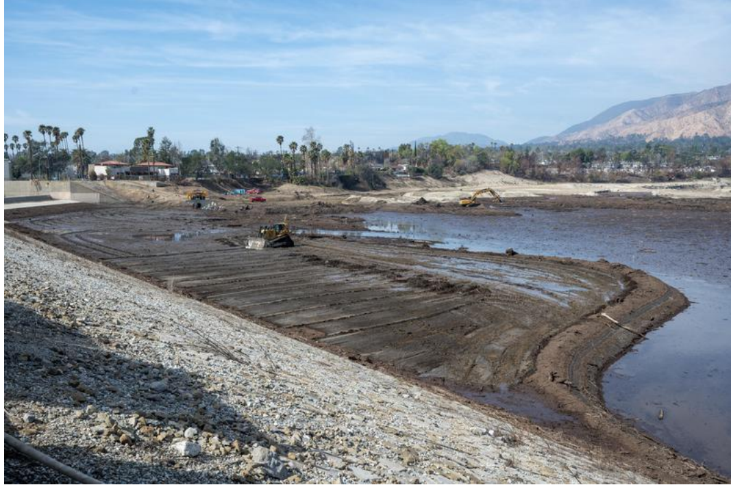
Photograph of post-Eaton Fire debris flow at Eaton Wash Dam
