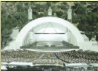
A view of the Bowl after project is completed.
