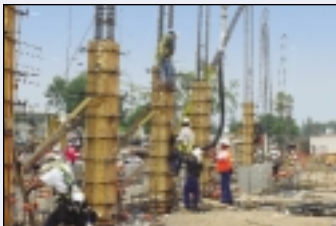
Construction, Los Padrinos Juvenile Hall Housing.
