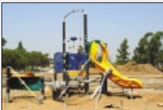
East Los Angeles Civic Center Renovation.
