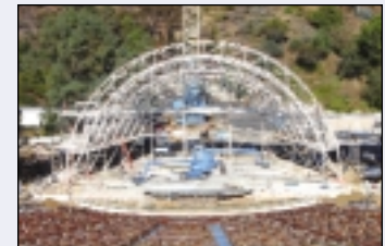
Hollywood Bowl Shell Rehabilitation Project.
