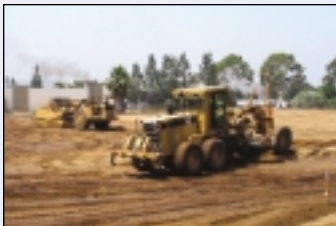
Grading, San Dimas Sheriff Station.
