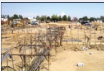
Construction, San Dimas Sheriff Station.
