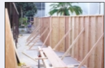
Construction, Santa Monica Courthouse.
