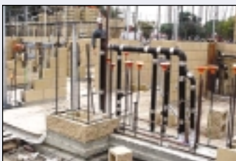
Construction, Jesse Owens Park.
