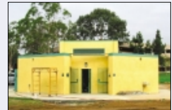
East Los Angeles Civic Center Renovation.
