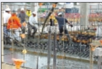
Construction, Los Padrinos Juvenile Hall Housing.
