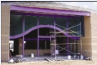
Construction, Jesse Owens Park.
