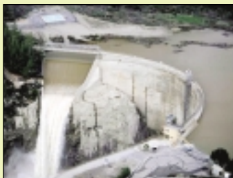
Water spills out of Big Tujunga Dam during 2005 winter storms.
