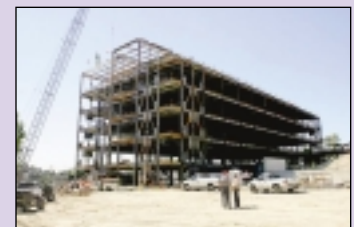
Construction is under way on the new crime lab.
