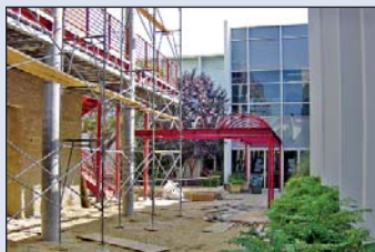
Santa Monica Courthouse
