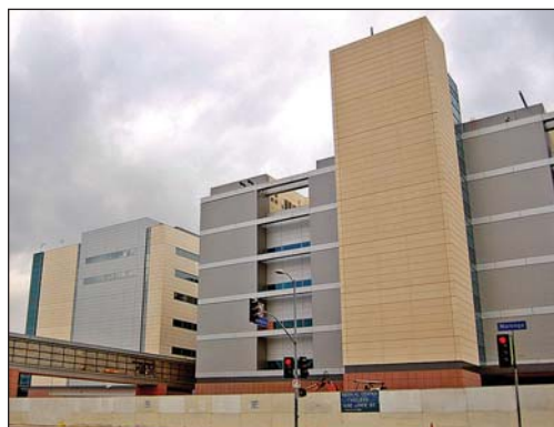
LAC+USC Medical Center Replacement Project under construction.
