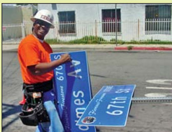
Employee Sterling Butler installs street name sign in Florence-Firestone area.
