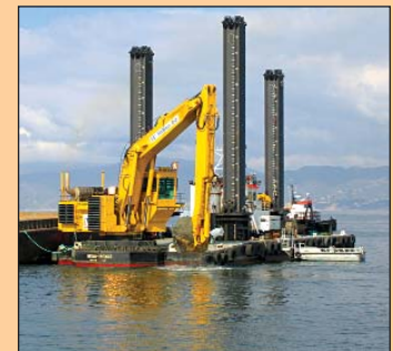
Marina del Rey dredging.
