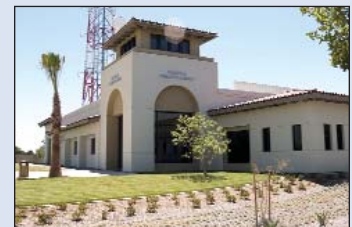
Palmdale Sheriff Station
