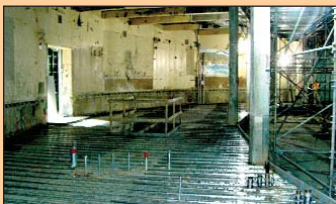
Mark Taper Forum lobby during construction.
