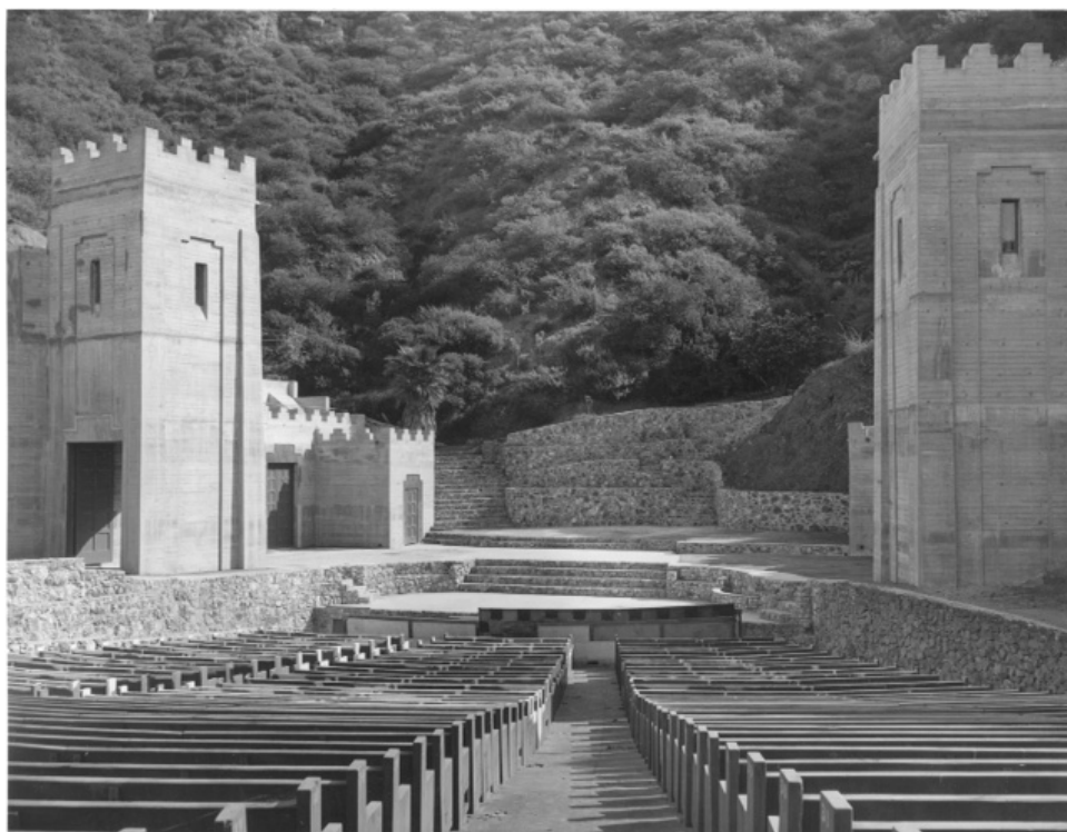
Figure 8 - By 1947 the lower stage was replaced and the stage towers were constructed. It appears that the retaining walls and staircases were reconstructed, as the landscaping and set piece are gone. Source: Los Angeles County Music Center.
