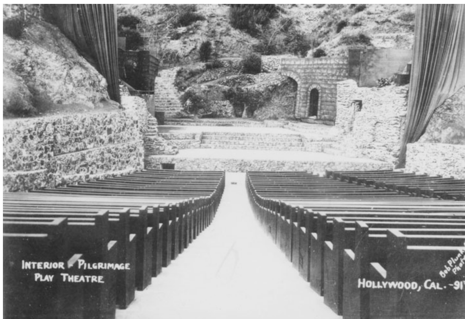
Figure 7 - The stage in 1931 included three levels. The lowest level appears to have had a concrete slab with stonework along the front. The staircase on the north appears to circle around to a part of the set to the south. Source: Los Angeles Public Library Photographs Collection.
