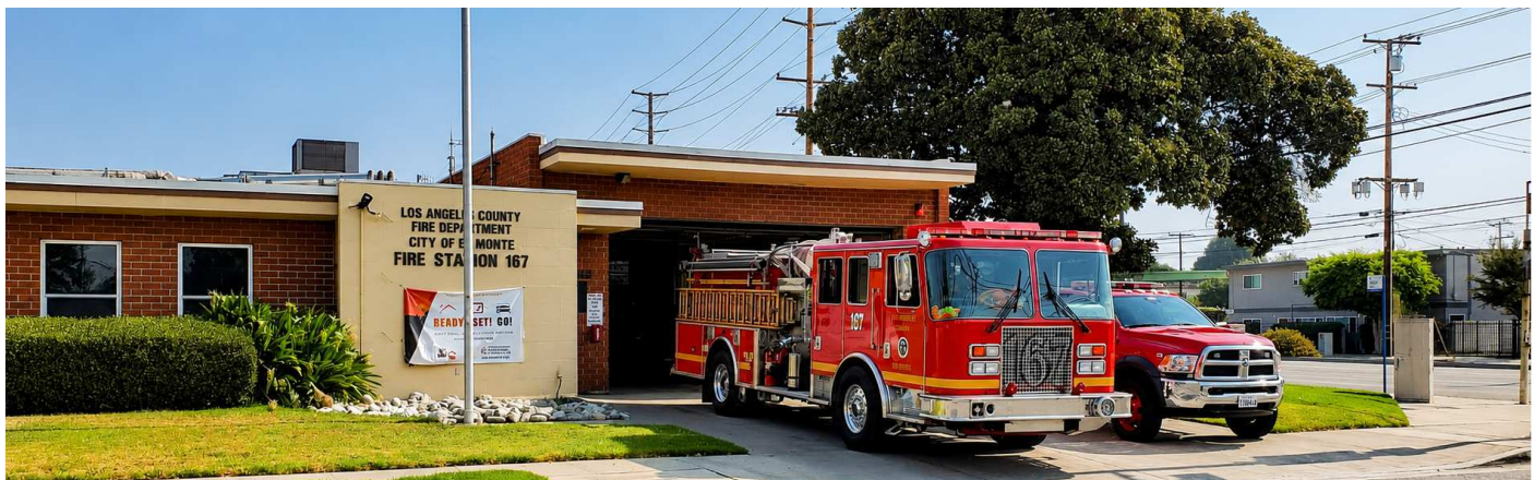
Fire Station 167, one of the stations supporting LA-DROP's planned expansion into eastern Los Angeles County.
