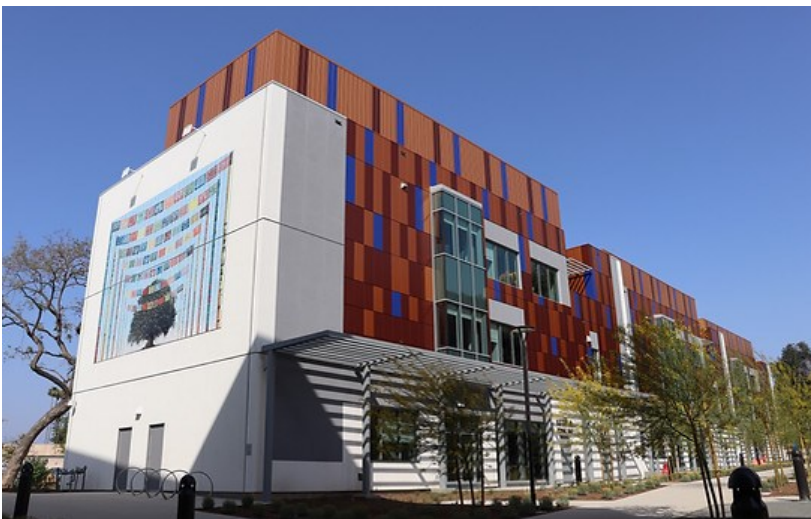
New Construction of the Restorative Village
