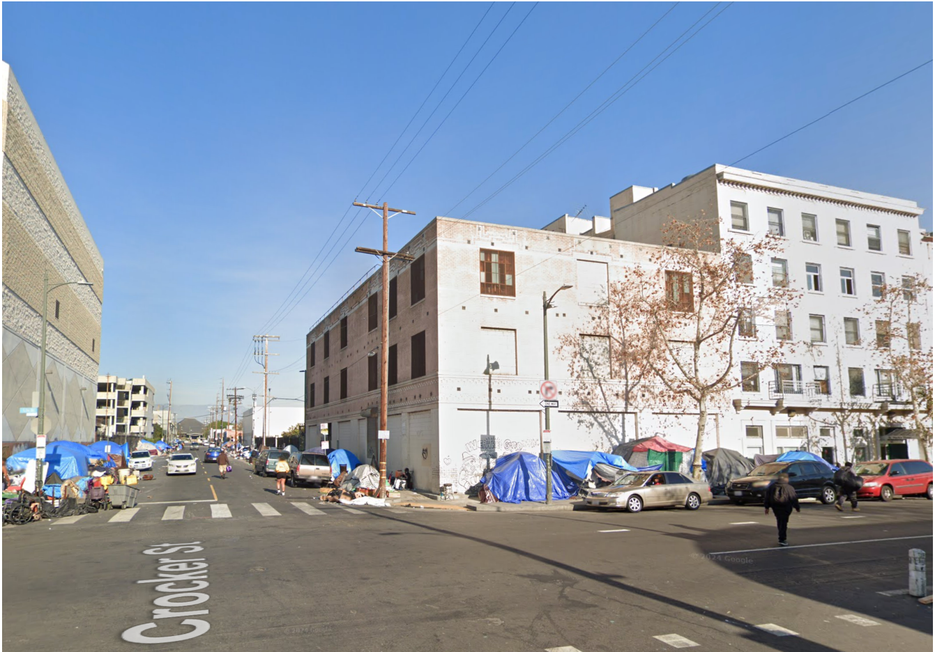
Figure 2: Project Site Existing Building (looking North along Crocker Street)
