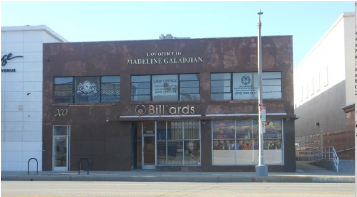
12135 Victory Boulevard, south elevation
