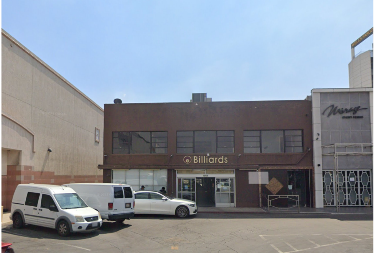
Figure 3: Project Site Existing Building (from Parking Lot in Back)
