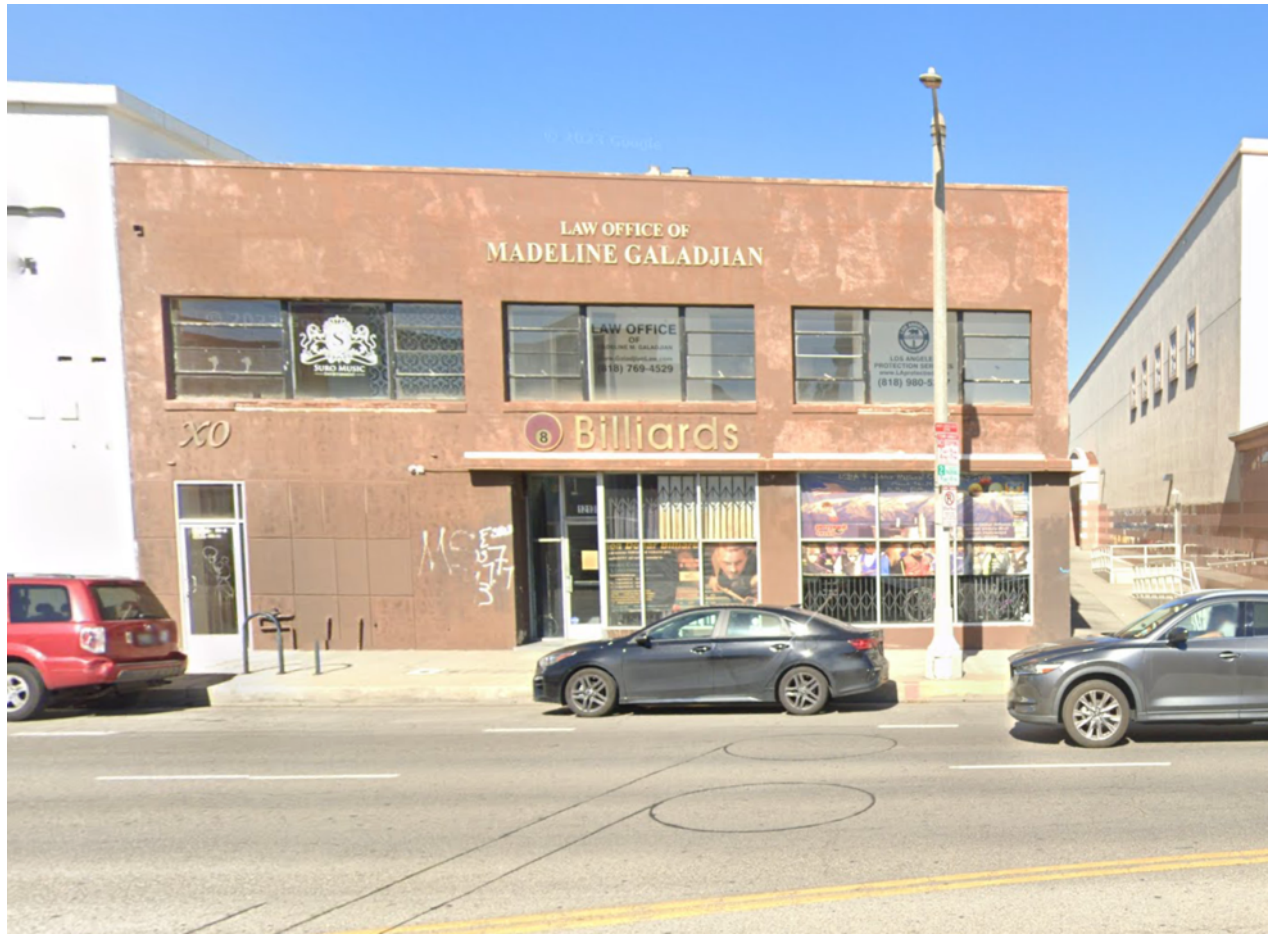
Figure 2: Project Site Existing Building (from Victory Boulevard)
