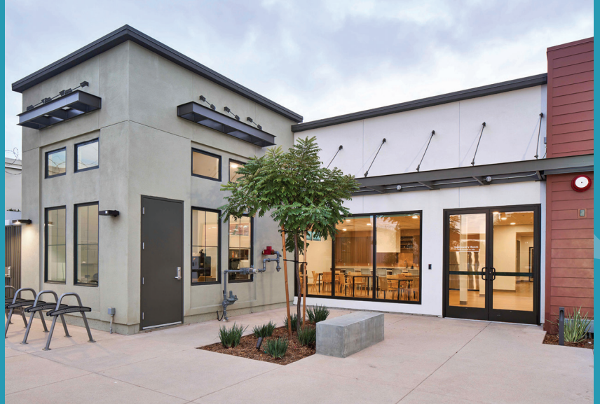
An outside view of Sagepointe, a 56-unit Permanent Supportive Housing community in Wilmington operated by Linc Housing, specifically for seniors 55+ who have experienced homelessness.
