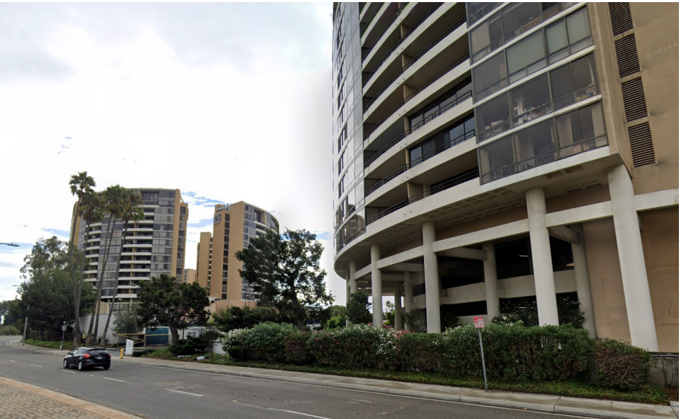
Existing Condition: View 2
