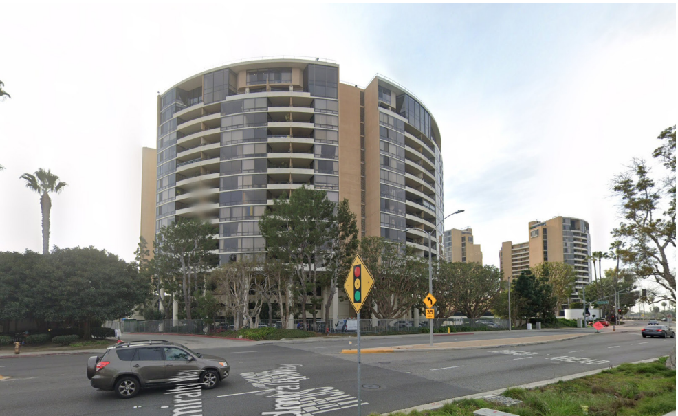
Existing Condition: View 1
