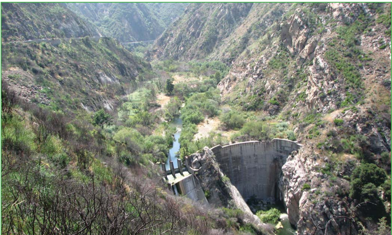
Rindge Dam, June 2008. The construction of the dam in 1926 led to the trapping of about 780,000 cubic yards of sediment behind it as shown in the photograph.
