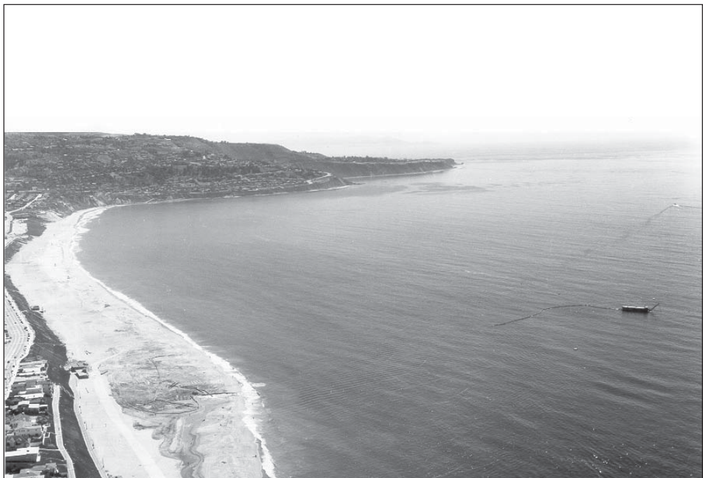
Nourishment of Redondo and Torrance Beaches in 1968. The 1.4 million cubic yard project is one of the most successful beach nourishment projects in the United States. The photograph shows the hydraulic dredge pumping sand onshore from the offshore under water borrow site.
