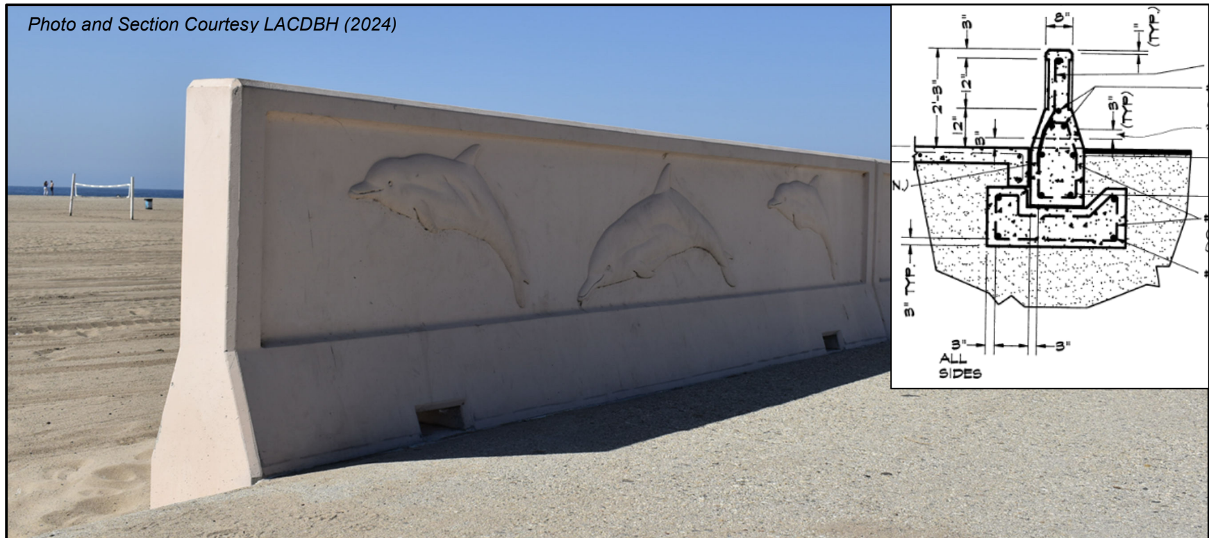
Figure 4-10. Photo and Cross Section of Low Sand Barrier at Zuma Beach
