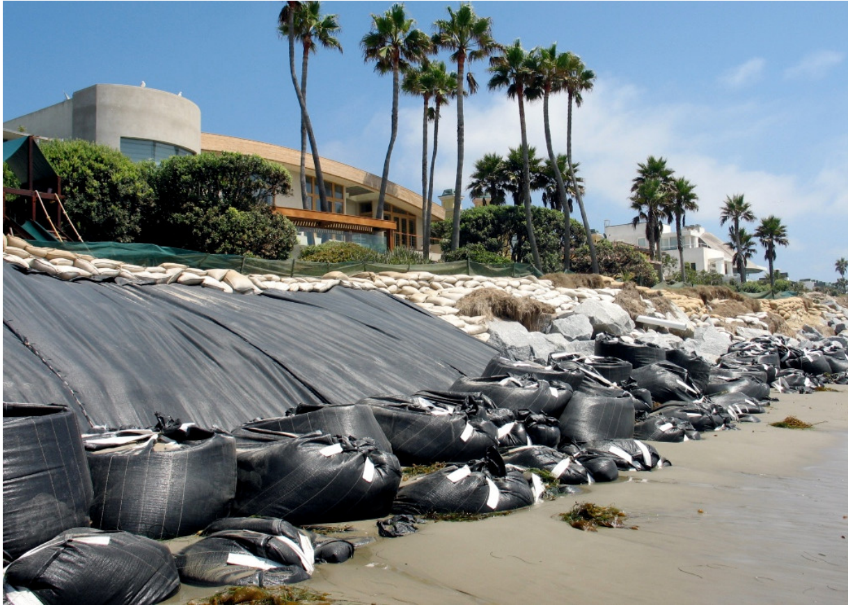
Figure 6. Sandbags were placed along the western end of Broad Beach in 2008.
