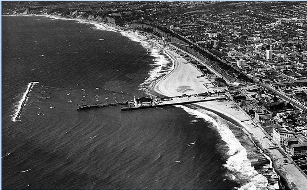
Santa Monica Breakwater (ca. 1937) Water and Power Associates
