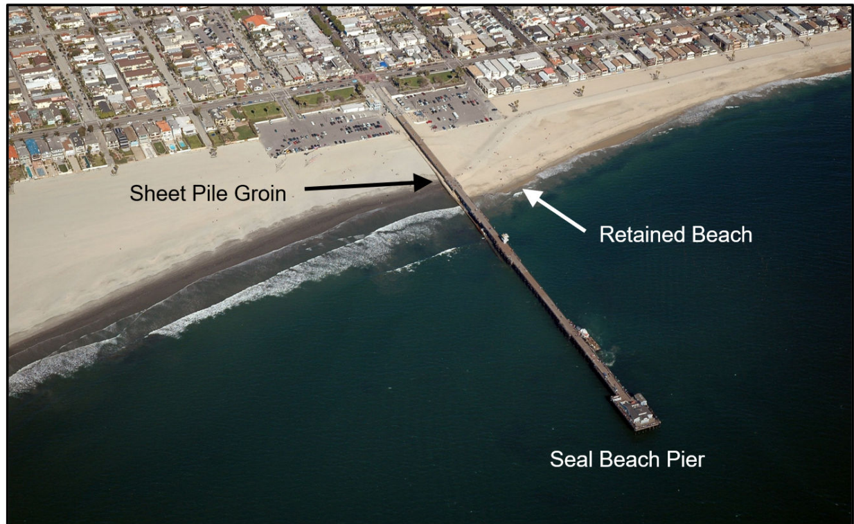
Figure 4-14. Beach Retained by Sheet Pile Groin at Seal Beach Pier
