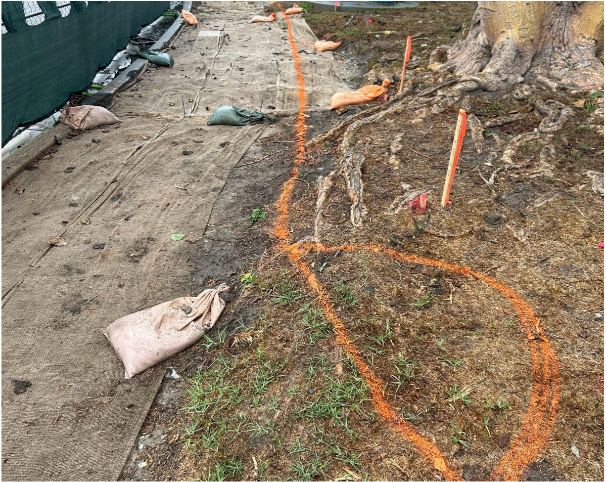
Area around VM-41 that will need hand excavation to determine root pruning options
