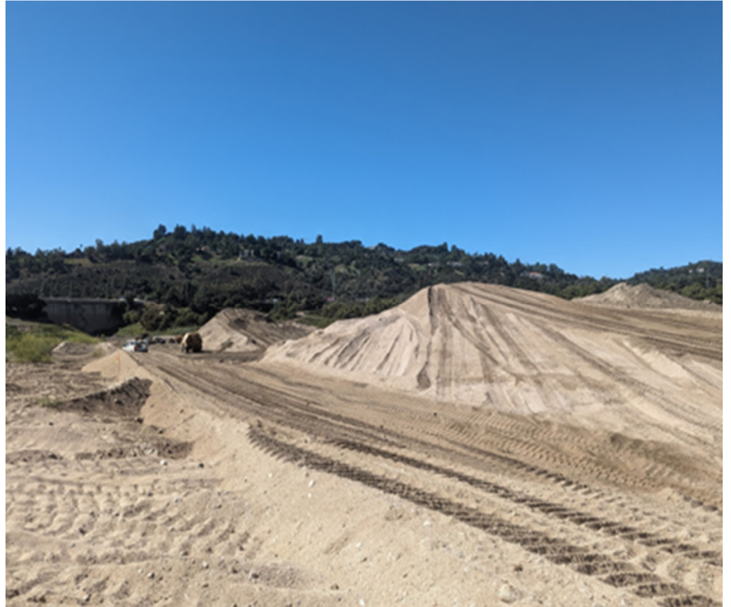
Sediment at Devil's Gate Reservoir
