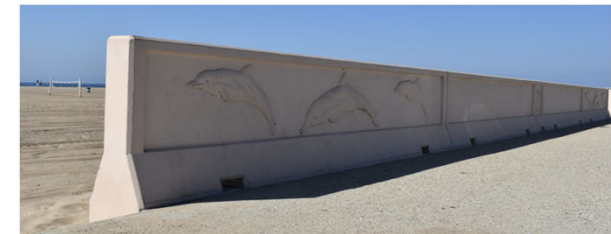
Example: K-rail barrier at Zuma Beach
