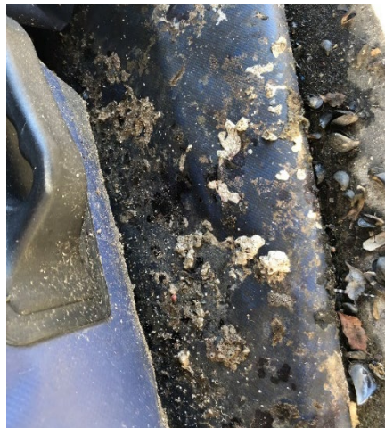
Figure 5: Fouling Under FAB Dock #2
