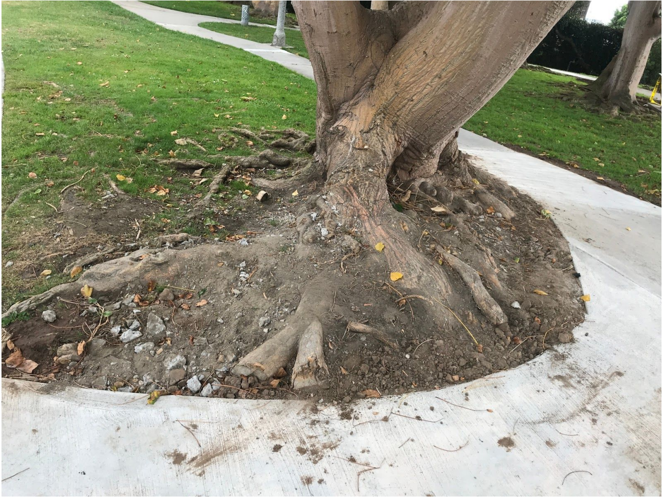
Photo 3 – Tree VM-30, large structural roots (>3”) being pruned more than 50%.
