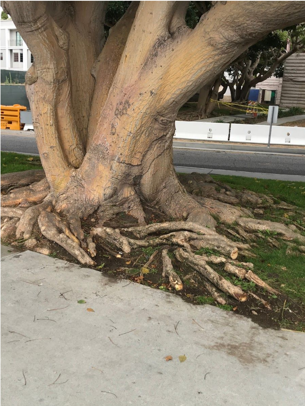
Photo 2 – Tree VM-28, Large structural roots (>2”) being pruned for new construction to sidewalk.
