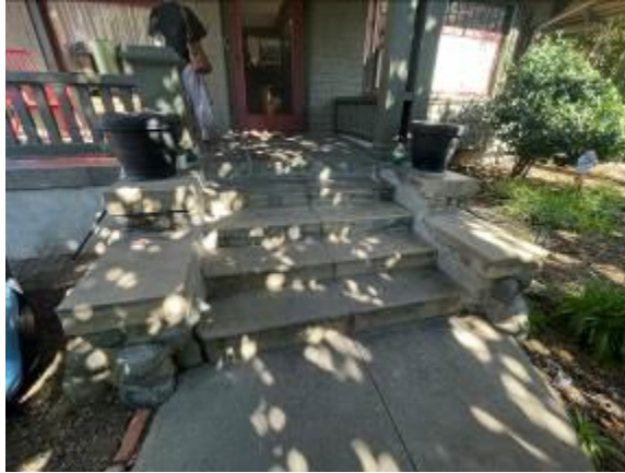
Figure 4. Detail of Entry Porch, Primary Façade (cast concrete steps accented with arroyo stone and cast concrete porch deck) SOURCE: Sapphos Environmental, Inc., 2023
