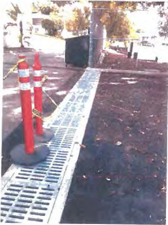
Trench Drain between New West AC Parking and Existing Sheriff's Station AC Parking
