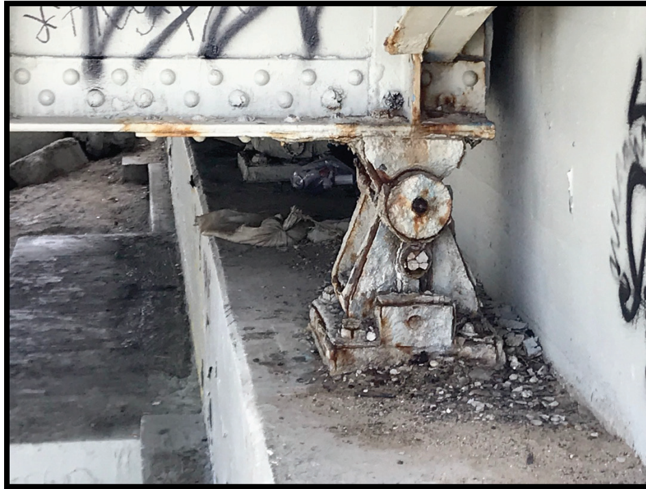
Figure 14. Original Construction Detail – Pacific Avenue Bridge
