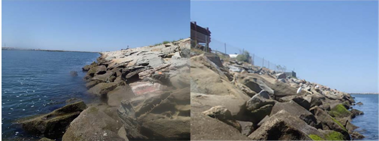
Figure 5. Upland area consists of rip rap revetment with and without concrete fill. Left image is north jetty looking downstream; Right image is south jetty looking downstream.
