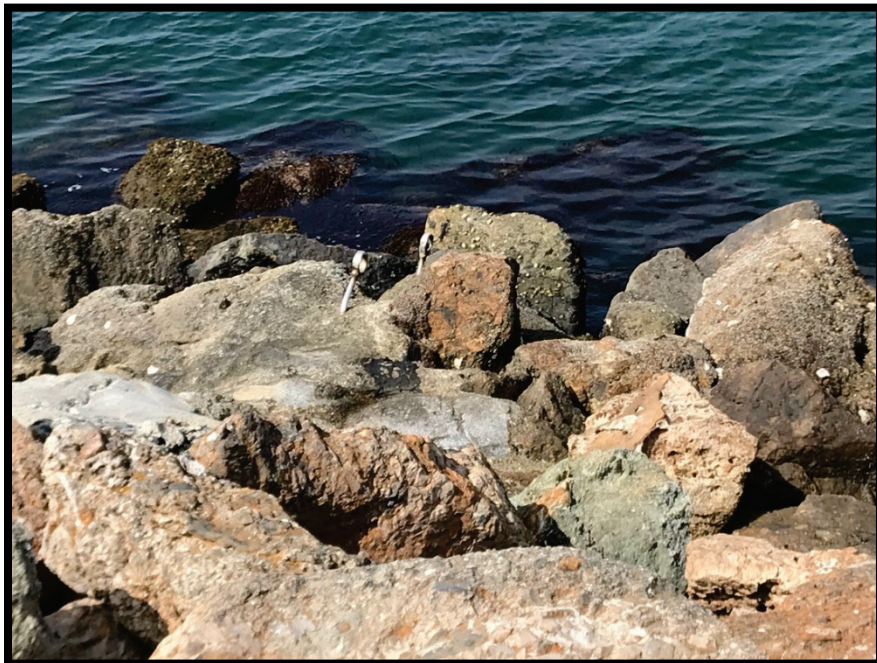
Figure 9. Rock, Concrete, and Existing Anchor Ties at Ballona Creek South Jetty
