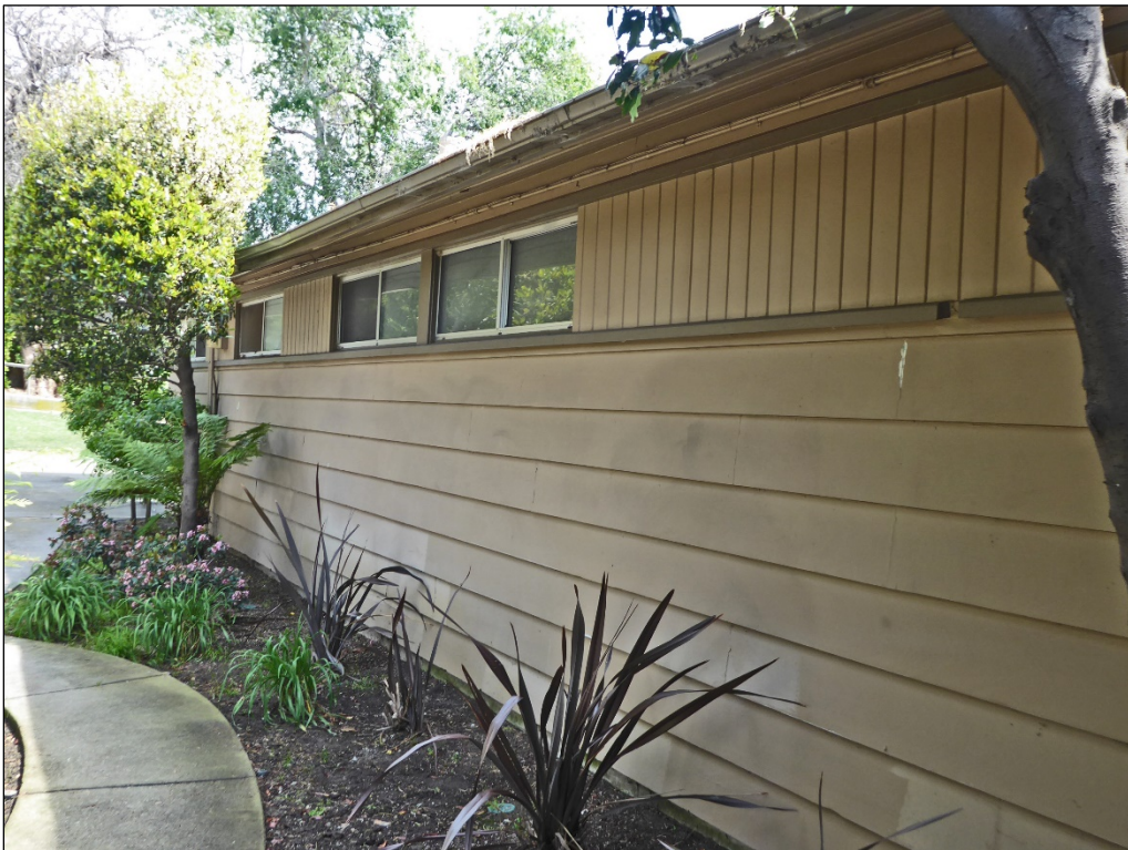
Figure 17. Exterior siding of Pro Shop.
