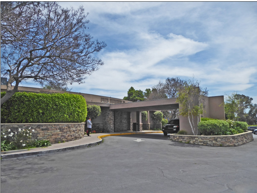
Figure 13. The porte-cochère at the primary entrance of the Clubhouse.
