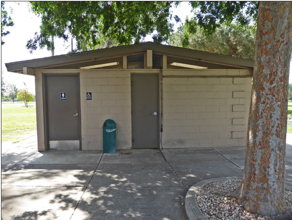
Figure 19. Comfort Station No. 2, entrance to women's restroom.
