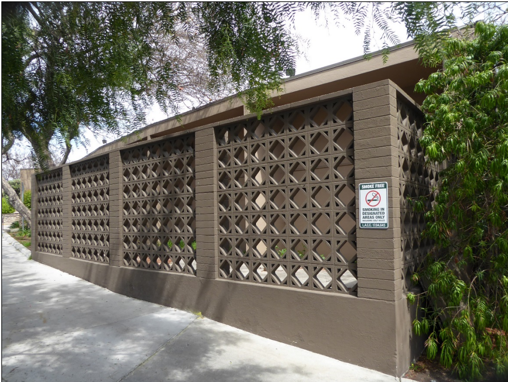
Figure 26. Patio with concrete-block screen.
