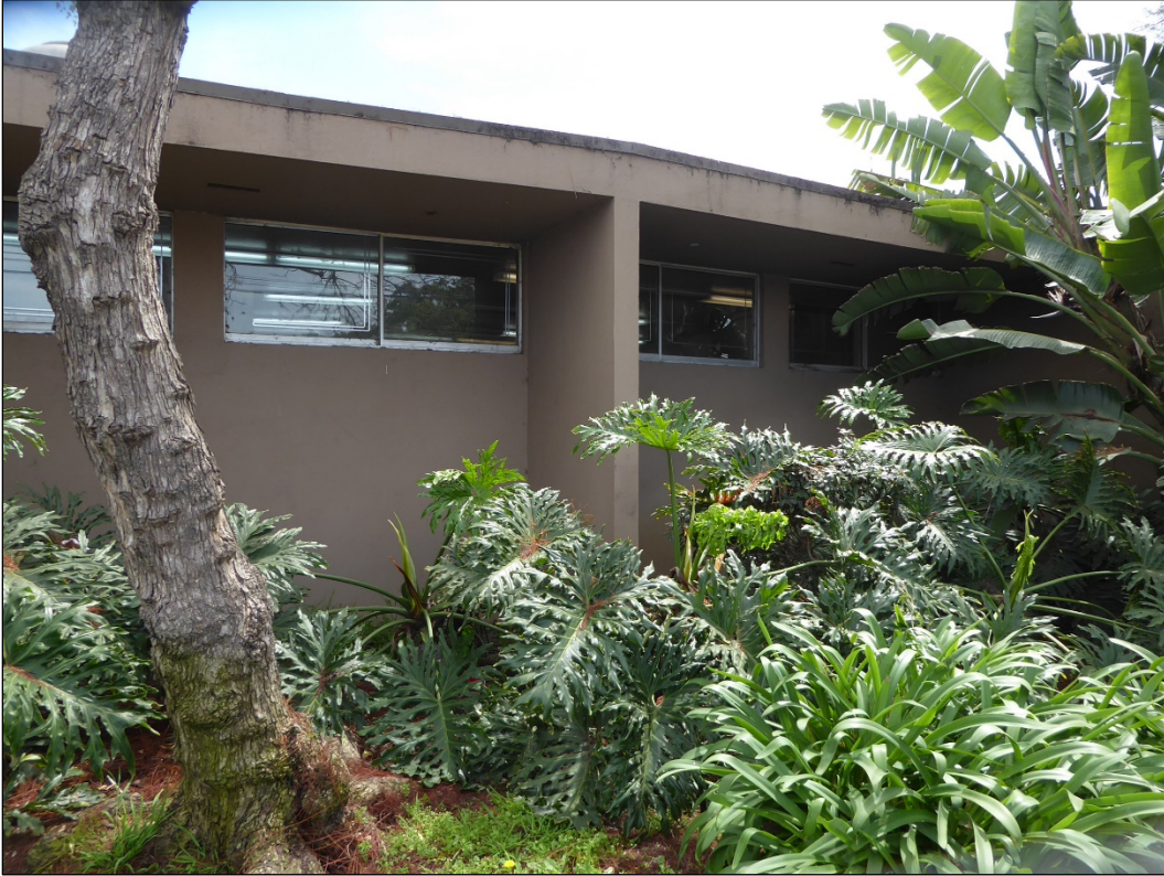
Figure 12. Vertical wall extensions at convex side of Clubhouse.
