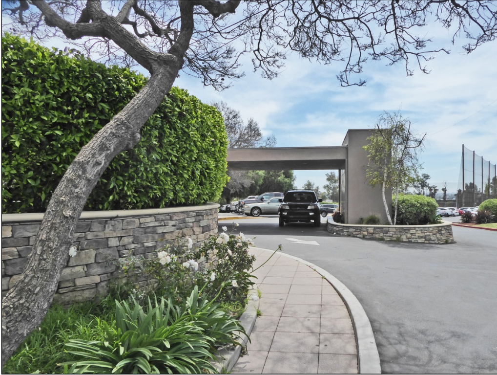
Figure 25. Patio with curved pony wall.
