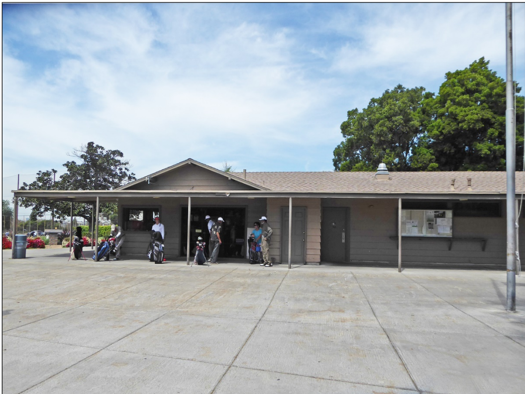
Figure 15. Pro Shop, view toward the primary entrance.
