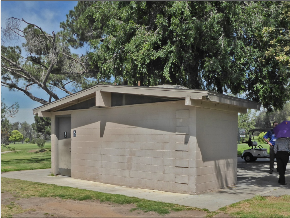
Figure 20. Comfort Station No. 2, entrance to men's restroom.
