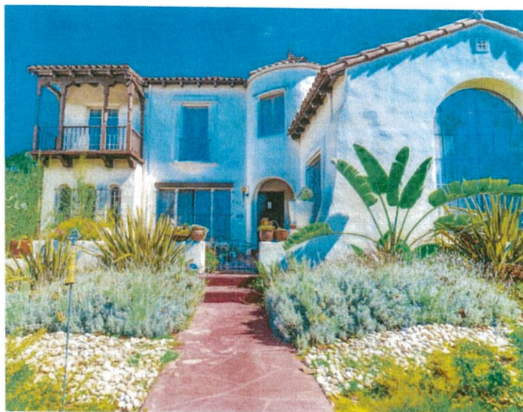
Figure 7. View toward the south of the north (primary) façade.
