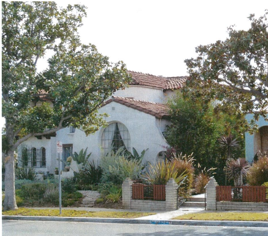
Figure 9. View toward the southeast of the north (primary) façade. Source: ASM Affiliates: Date: December 3, 2015.
