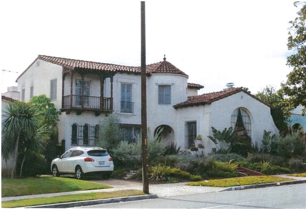
Figure 8. View toward the southwest of the north and east facades. Source: ASM Affiliates: Date: December 3, 2015.
