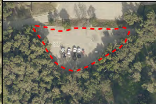
Temporary District Operations Trailer Area
