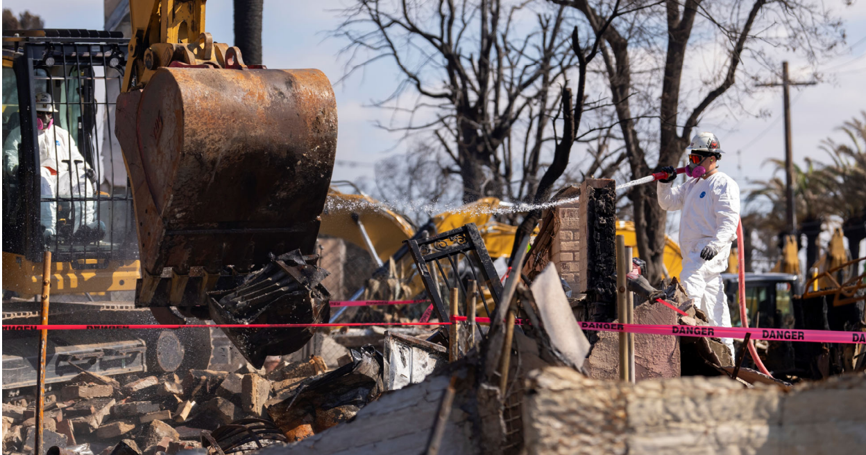
Figure 39: Debris Removal in Altadena
