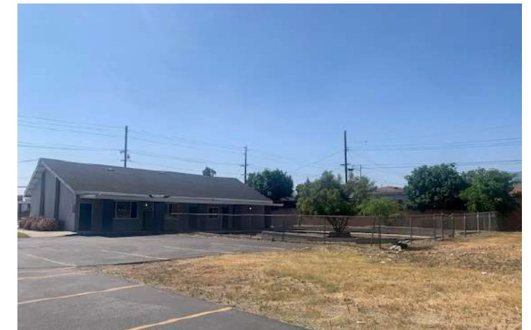
⑤ VIEW FROM PROPERTY. - FACING EXISTING STRUCTURE
