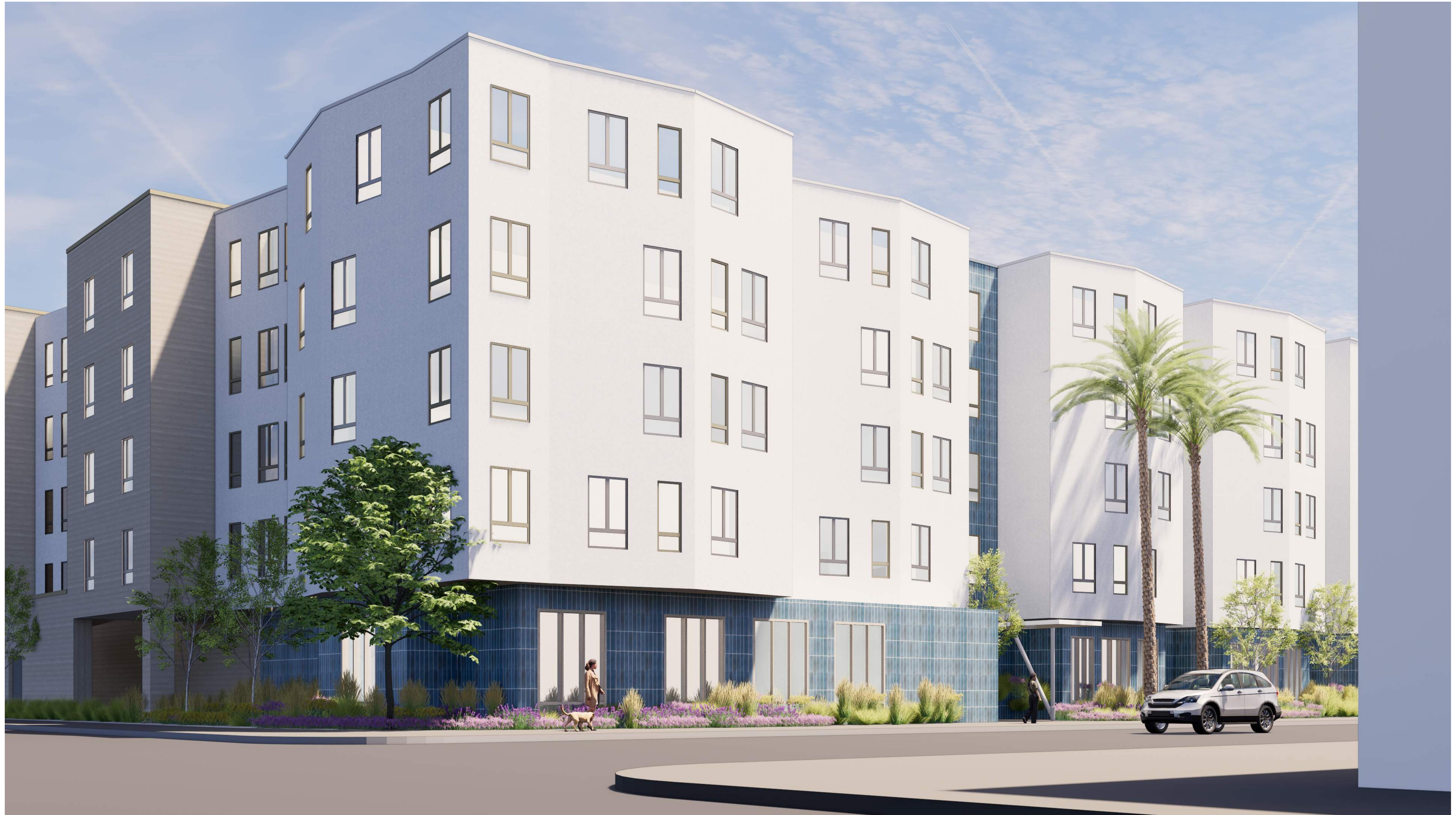
CORNER OF ELM AVENUE AND 36TH STREET
