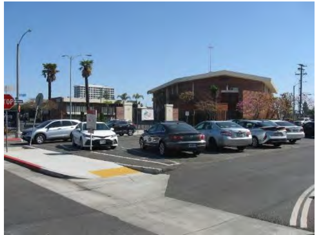
Another view of Grace Church across East 36 th Street
