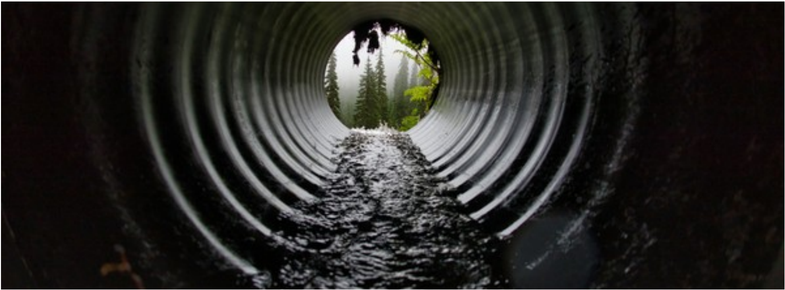
Data center construction is posing new concerns for local wastewater utilities. Marco Bicca/Unsplash
