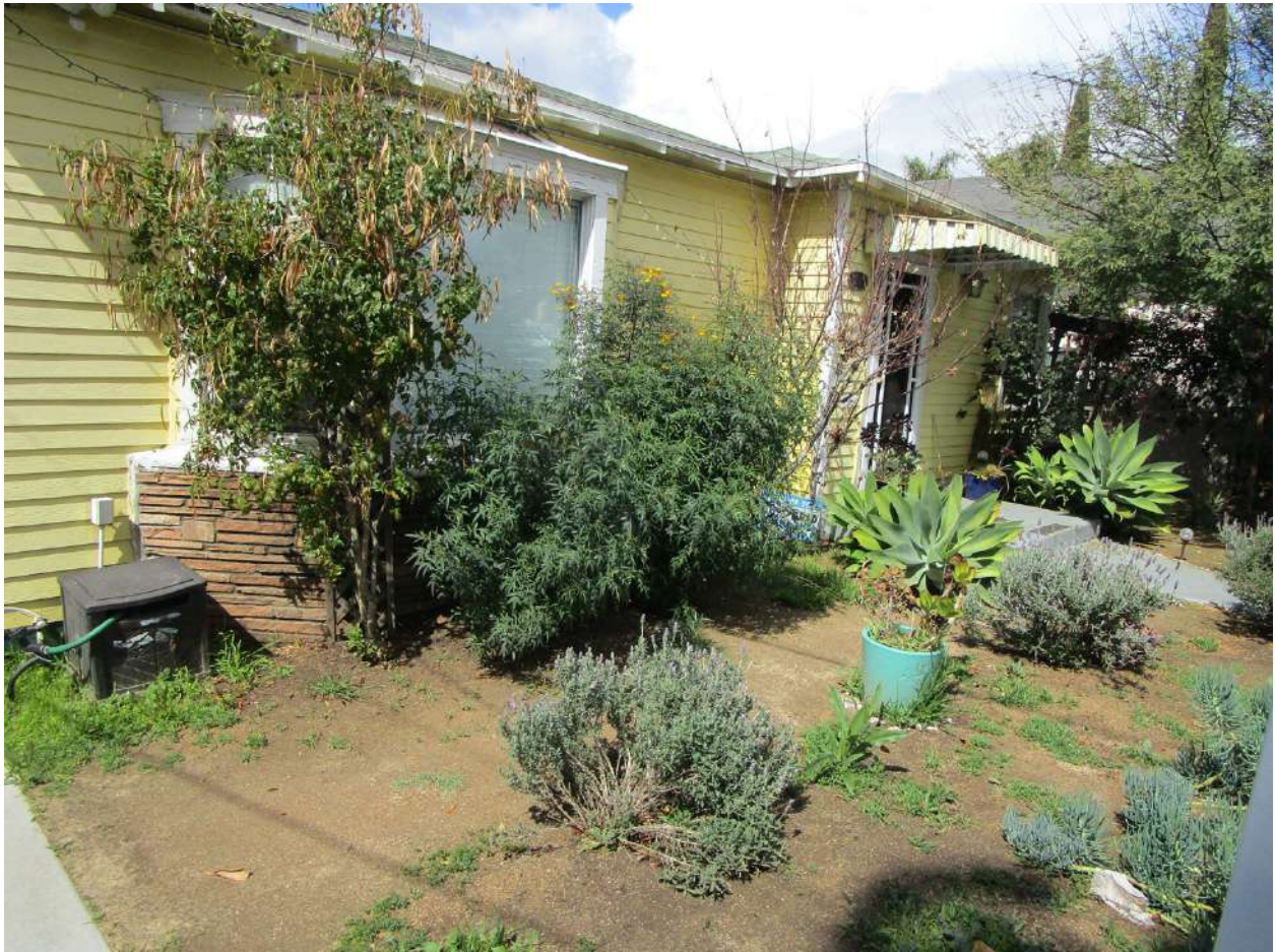
Photograph 10 exterior-207 S. Boyle
