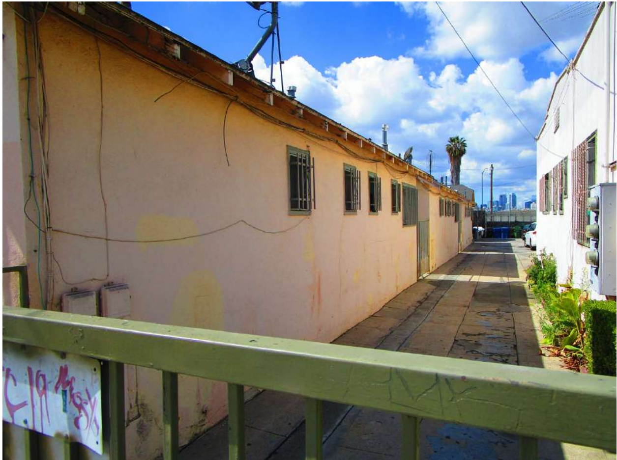
Photograph 22 exterior 133-139 S. Boyle
