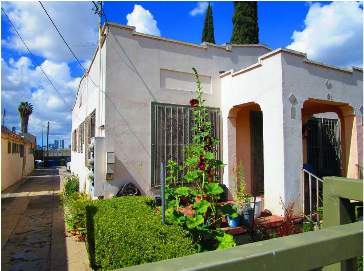
Photograph 21 exterior 133-139 S. Boyle
