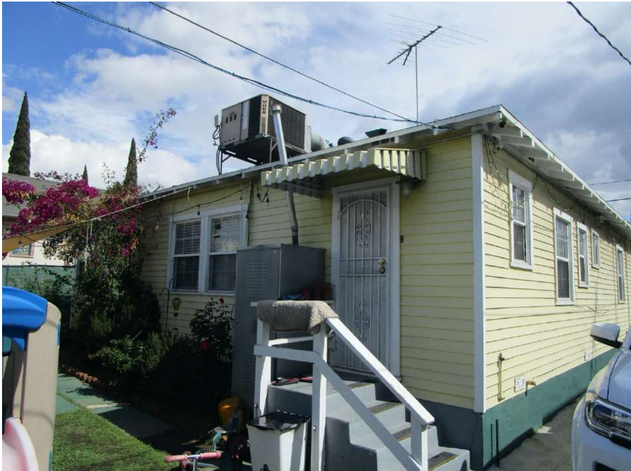
Photograph 11 exterior-207 S. Boyle
