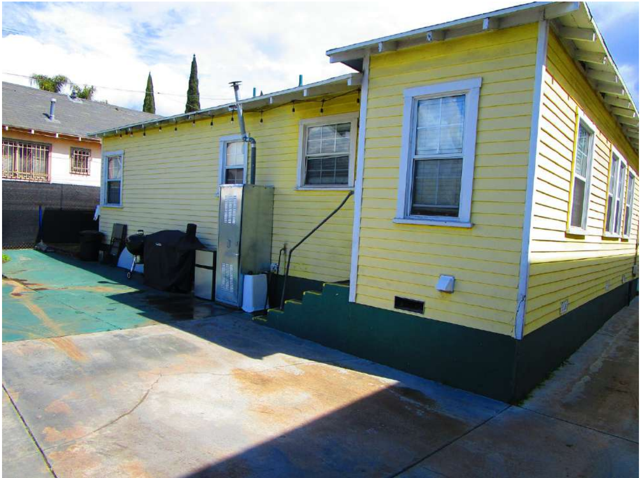
Photograph 13 exterior-207 S. Boyle
