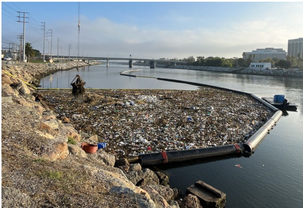
Figure 2: Los Angeles River trash boom
