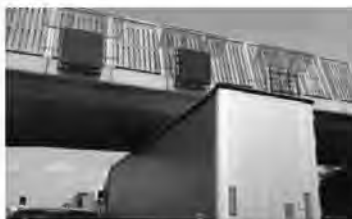
Figure 5.6. In the Netherlands, walls were designed to avoid light trespass from a highway to a wildlife bridge with commuting routes (© H. LIMPENS).
