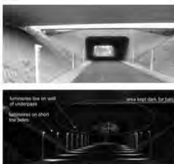
Figure 5.3. Installation of luminaires on short poles for mitigating the effect of ALAN on a commuting route through an underpass in the Netherlands (the same place in daylight and at night). This solution was proven as efficient for P. pipistrellus but not for the low-flying species M. daubentonii (© F. BREKELMANS).
