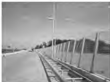
Figure 5.7. Partially shielded noise screens, installed during the construction of a new motorway in the Netherlands for avoiding light trespass to a compensation area with bat habitats (© V. I. OER).
