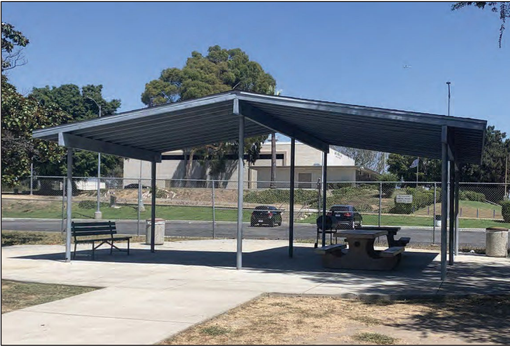
Looking south to picnic area.
