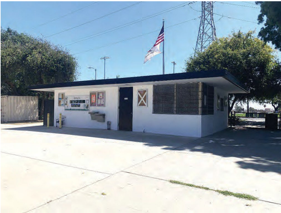
Looking south to office building.
