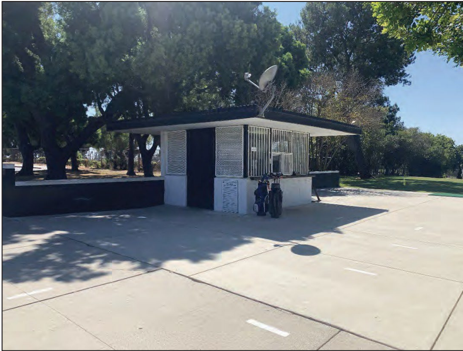
Looking southwest to concession stand.
