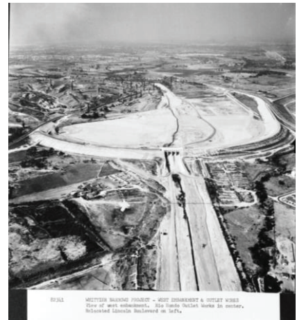
Whittier Narrows Dam under Construction, 1950 (Source: Los Angeles Public Library)
