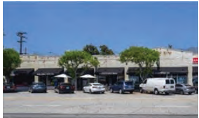
835 Mariposa Street, Altadena AIN: 5845017014 Date of Construction 1924
