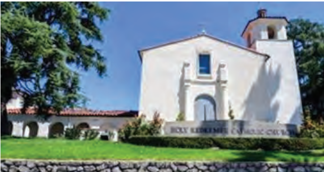
Holy Redeemer Catholic Church 2411 Montrose Avenue AIN: 5807001030 Date of Construction: 1926/1928
