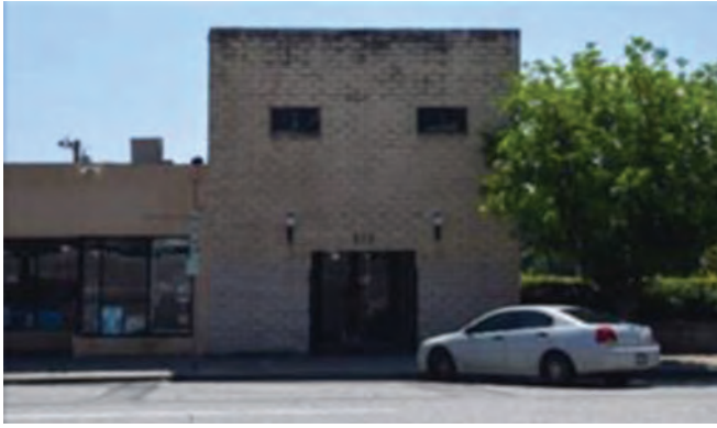
868 E Mariposa Ave, Altadena AIN: 5845018009 Date of Construction 1924
