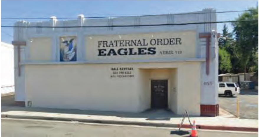
455 East Woodbury Road, Altadena Date of Construction 1940
