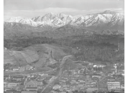
Construction of Pasadena Freeway, 1962 (Source: UCLA Libraries)
