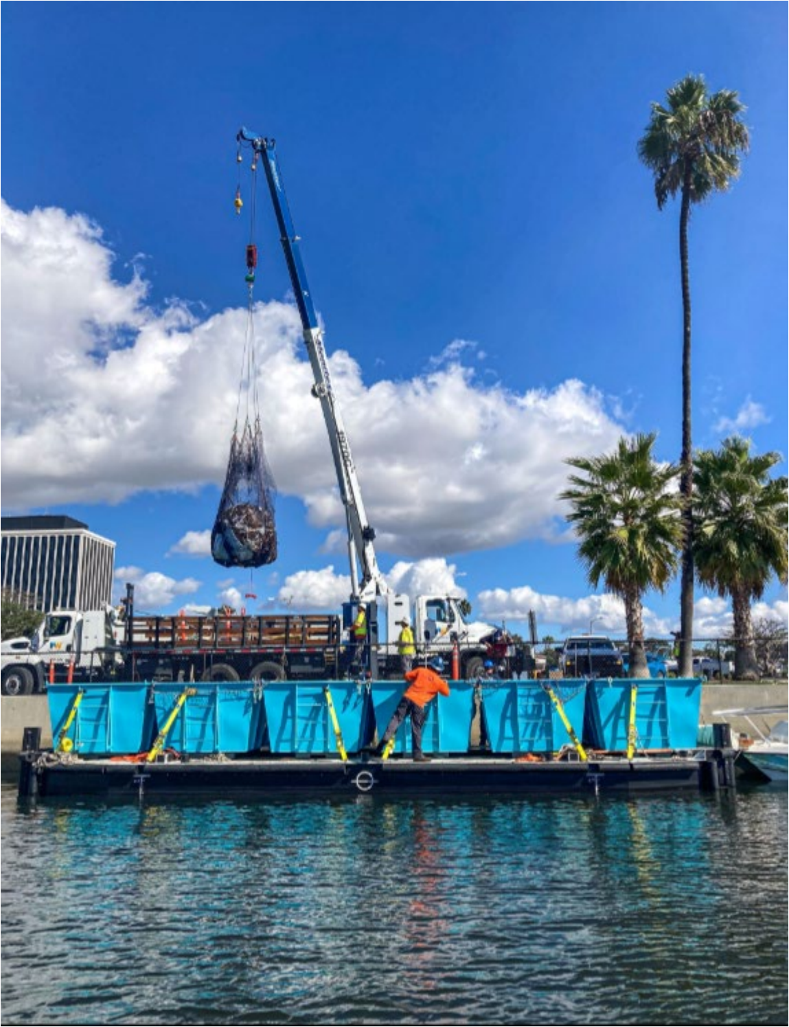
Figure 5 – Dumpsters and dumpster barge removed for trash disposal
