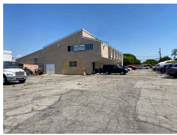
Two-Story Building On-Site
