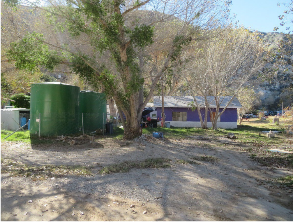
Photo #9-Water tanks/recreation room
