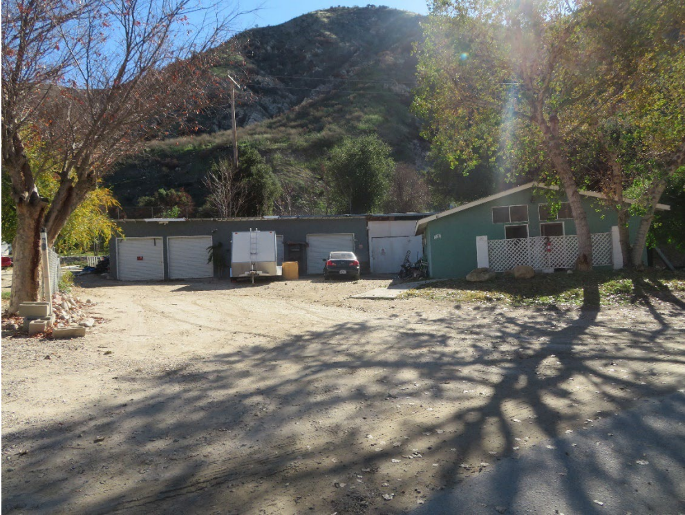
Photo #10-Maintenance building and east restroom building
