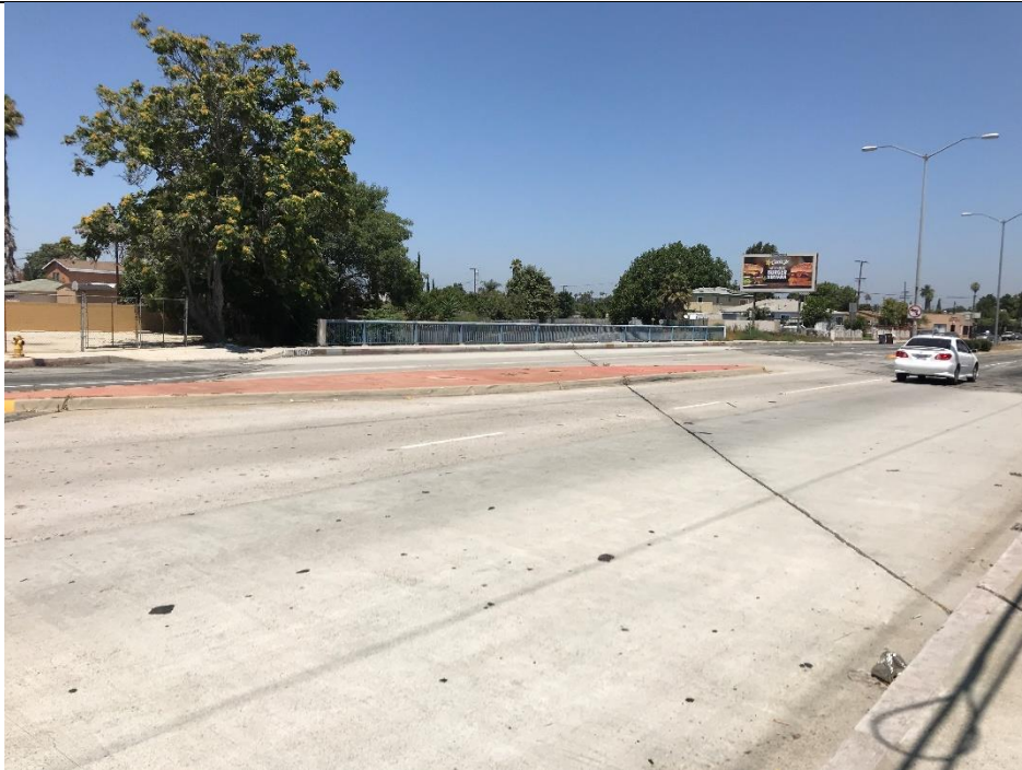
Facing northwest toward the Wilmington Avenue bridge deck.
