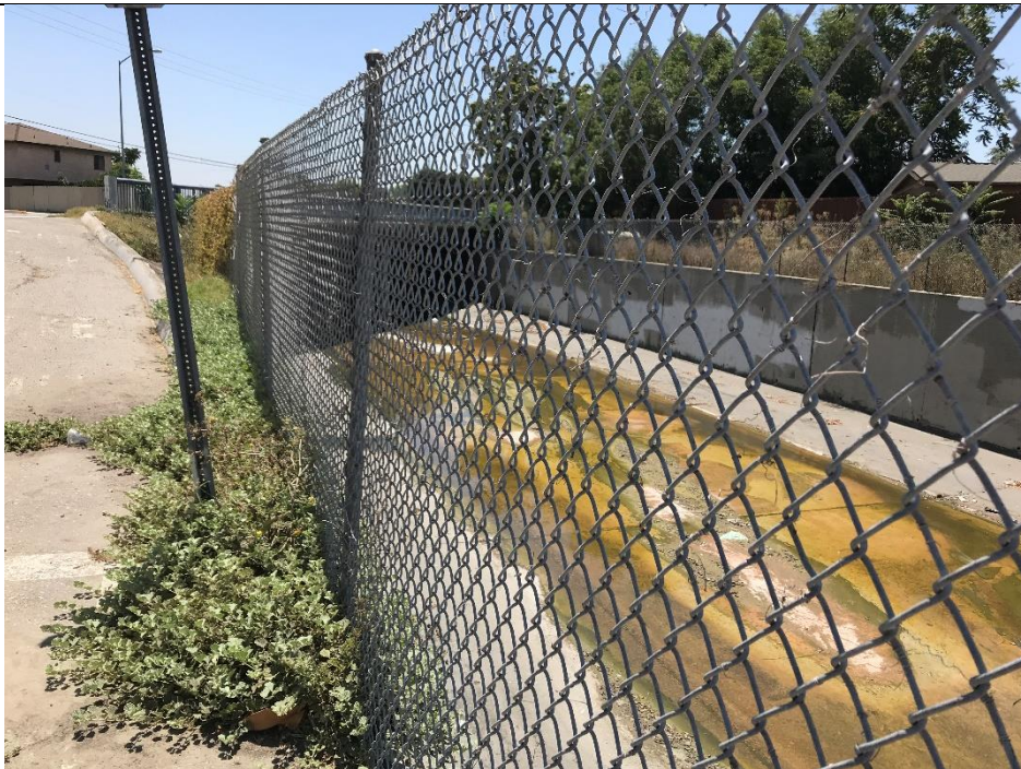
Facing southeast toward the western side of Wilmington Avenue bridge over Compton Creek.
