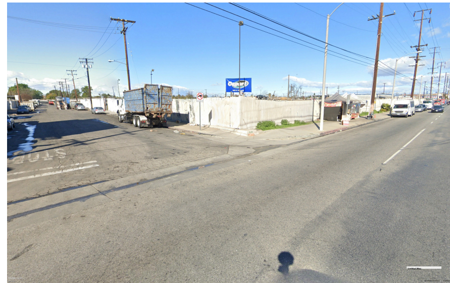
Figure 2 - View of Subject Property from Southwest corner.
