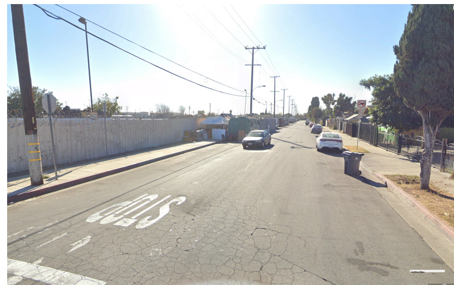
Figure 5 - View facing south down Lou Dillon Ave, Property on the left.
