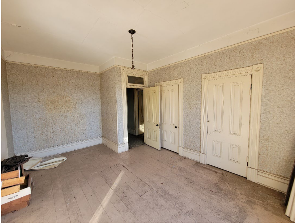
Photo 11 Second floor bedroom, view to southeast
