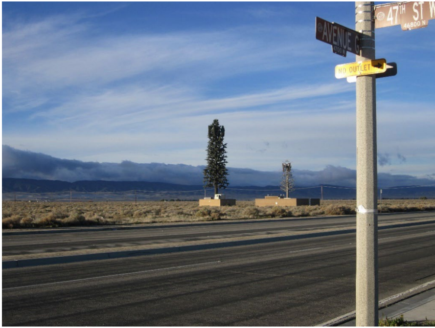
Cell towers in close proximity
