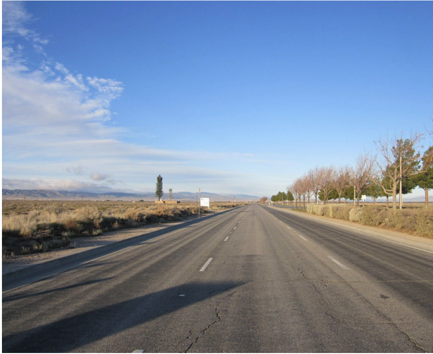
Additional view looking west from W Ave G with to right of photo. The road consists of three lanes in each direction in front of both of the subject parcels.
