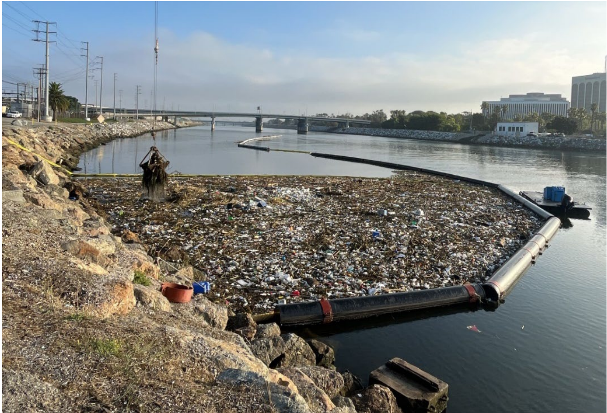
Figure 2: Los Angeles River trash boom
