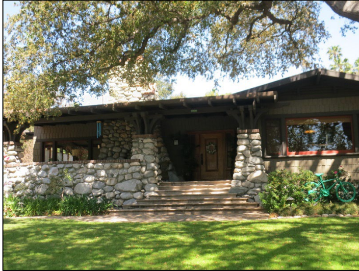
1115 E. Woodbury Road Historic Highlands Historic District Altadena
